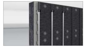
Apply joint tape on vertical bearing profiles
