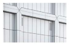
**Surface finishes.** The innovative HT surface coating prevents the formation of algae, moss and microbes while the self-washing effect ensures permanently clean facades.
