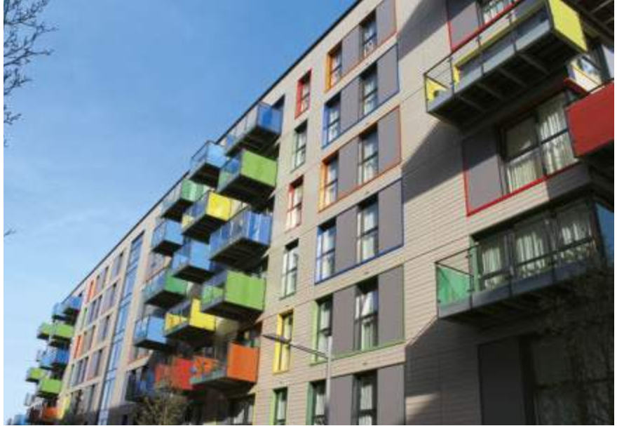
Hale Village Housing, Londres, Grande-Bretagne / Cartwright Pickard Architects / Achèvement 2012
